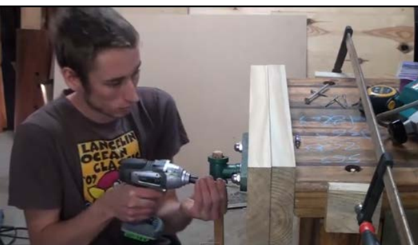
7. Screw front vice to handle end casting
